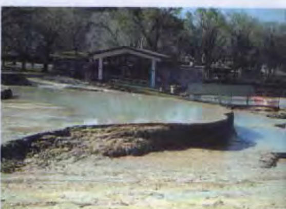
State Bathhouse, Hot Springs State Park, Thermopolis. Wyoming Travel Commission Photo
