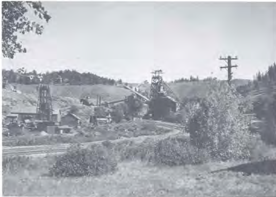
Figure 7. Colorado Fuel and Iron Company's Sunrise Mine in the Hartville Uplift. The mine has a rated annual capacity of approximately 600,000 tons. Hematite is mined from iron formations, and the ore is shipped to C.F. & I.'s blast furnaces in Pueblo, Colorado (Hausel, 1978). Photograph by W.D.H., 1980.
