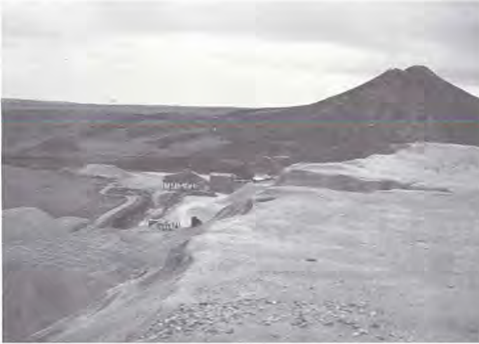
Figure 16. Great Western's Horse Creek property. Quarrying of this property began in 1912, and underground methods were initiated in 1926. The limestone occurs in two steeply dipping ( 80^{\circ} NE), massive beds that average 23 feet thick. The footwall is dolomite, the hanging wall a hard, massive red sandstone (Osterwald and others, 1966). More than four million tons of rock have been mined since 1912. Presently, five years of reserves are stored on the surface. Photograph by W.D.H., 1980.
