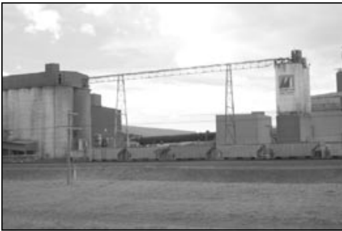
Figure 13. Mountain Cement's cement plant south of Laramie.
