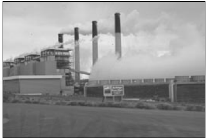
Figure 11. The Jim Bridger Power Plant about 30 miles east of Rock Springs consists of four 530-MW generating units fueled by coal mined at the nearby Jim Bridger Coal Mine. Photograph by Richard W. Jones.
