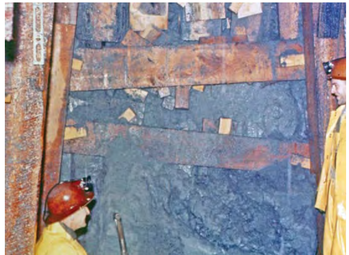
Figure 35. A9 Drift heading near south end after it had penetrated the water table. Water is dripping and running into the drift from the face, walls, back, and floors. In wet ground such as this, no face could be left open for more than a few minutes without caving, hence the breast boards shown in this picture. The vertical streaks scattered in the picture were caused by water dripping from the back. The drift at this point was being driven in unaltered silty sand. Photo by R. V. Bailey.
