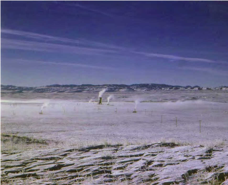
Figure 2. Shirley Basin Mine looking northeast toward the Laramie Range from Moss Agate Hill, February 1962. The temperature is well below zero and condensed moisture can be seen at the top of the head frame. The plumes from the small buildings are caused by exhaust moisture from heaters used to heat ventilation air for the mine. These two buildings are located at the surface site of cased escape-ventilation holes which intersect drifts underground. Photo by R. V. Bailey.
