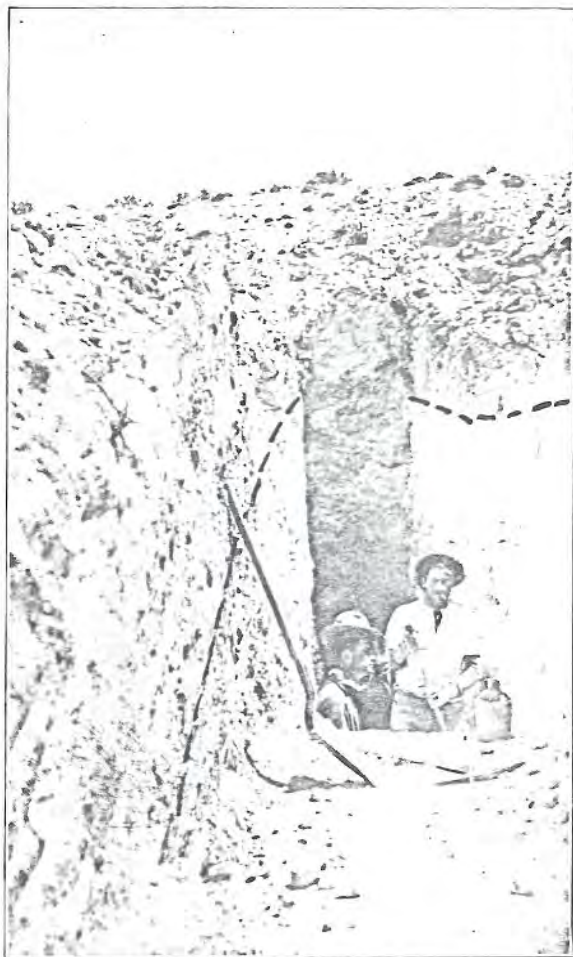
Shaft No 2. Through 15 feet of solid sulphur rock assaying 82%. Dotted line shows where sulphur commences.
