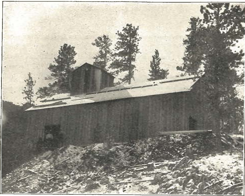
VIEW OF THREE CRIPPLES SHAFT HOUSE, NORTHEASTERN ALBANY COUNTY.
