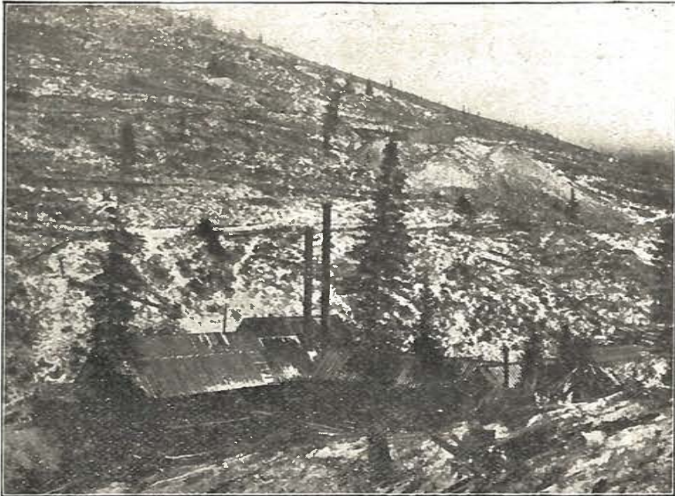
General View of Shaft and Tunnel House at the Doane-Rambler Mine, Southern Carbon County.
