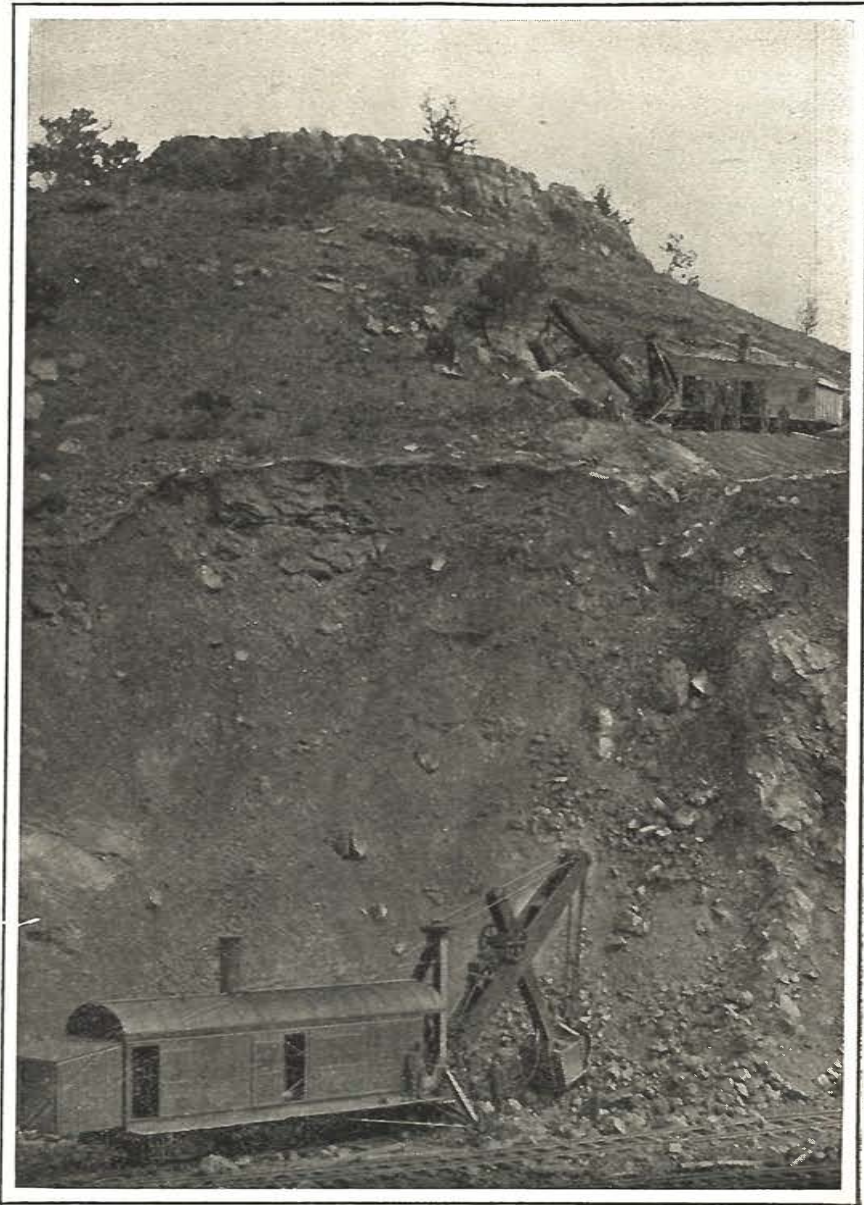
Part of the Sunrise Iron Mines of the Colorado Fuel and Iron Company, at Sunrise, in Northeastern Laramie County. The upper steam shovel is stripping off surface dirt and the lower shovel is loading iron ore.
