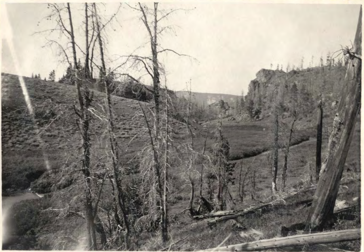
View looking northerly and down the "Neck" from a point on the Hawkeye Claim, showing the narrow condition of the river bottom at this point: the hydraulic works to be installed at a point opposite the high cliff at right of picture.
