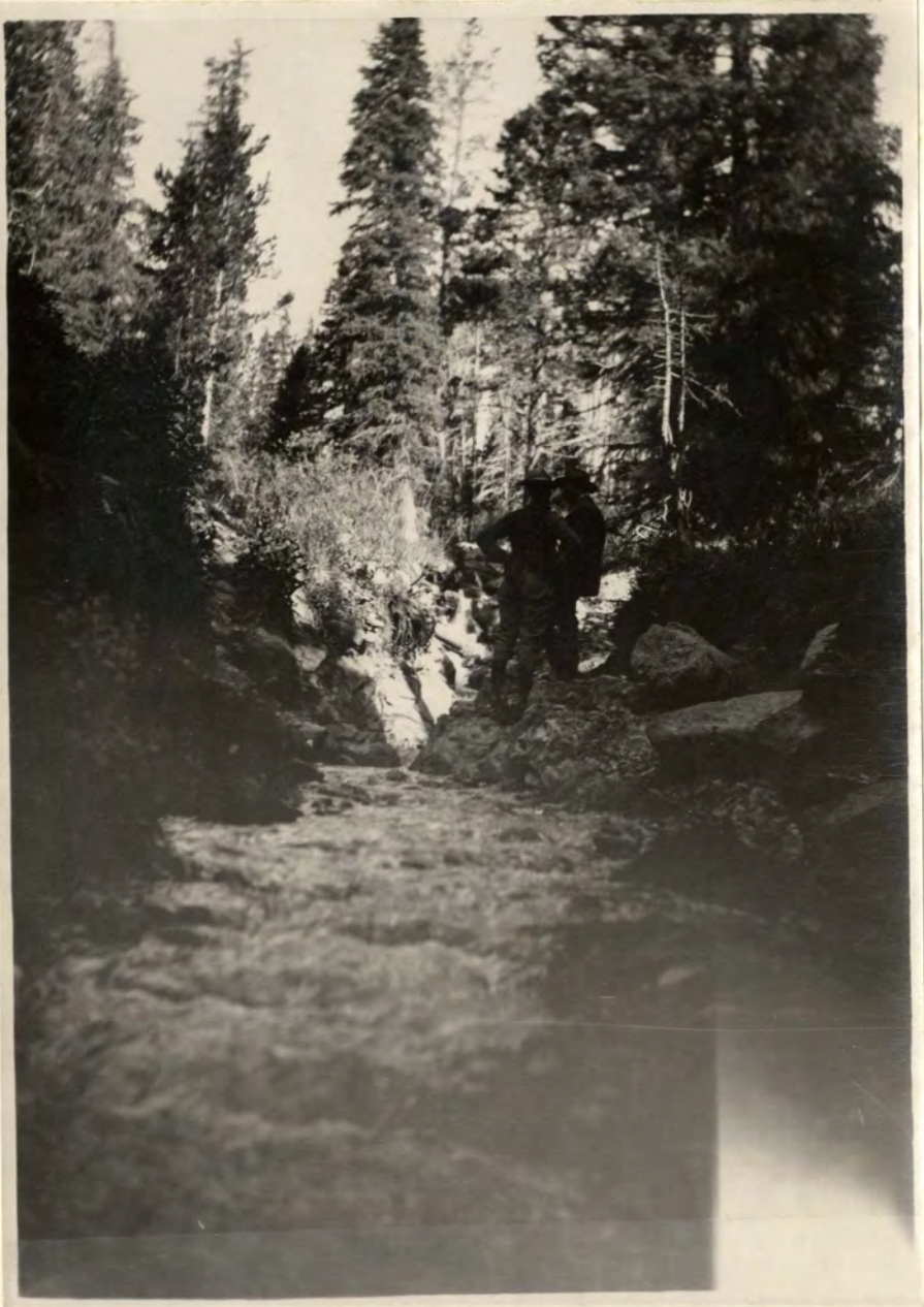
View on the Lafayette Claim looking westerly, showing the upper portion of the Lafayette Cut, where it is recommended that work be done during the present season?
