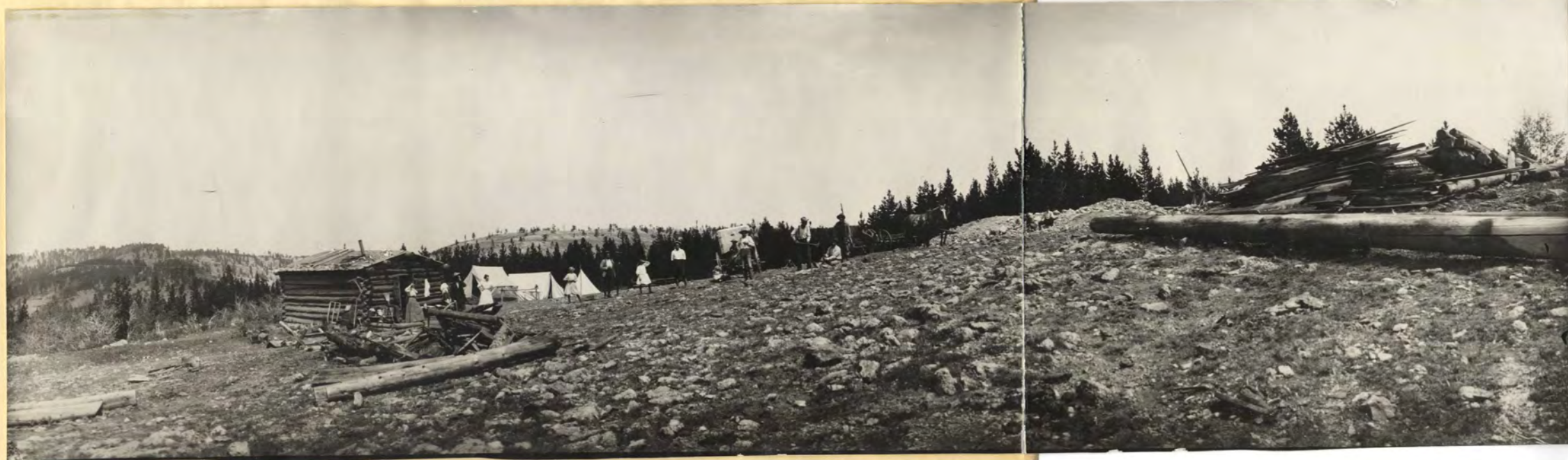
A view at the McConnell shaft, looking easterly from a point opposite the shaft and showing present camp and surface conditions.
