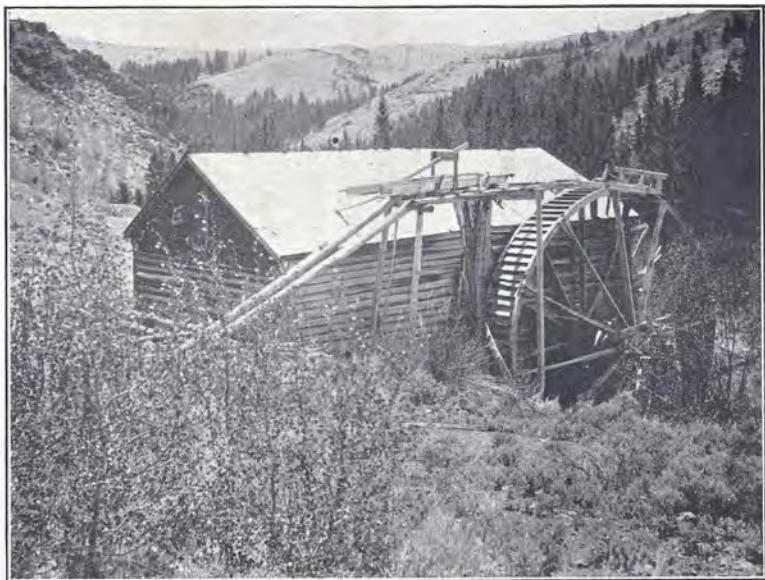
A. AN OLD TEN-STAMP MILL IN SOUTH PASS DISTRICT. Driven by 30-foot overshot water-wheel.
