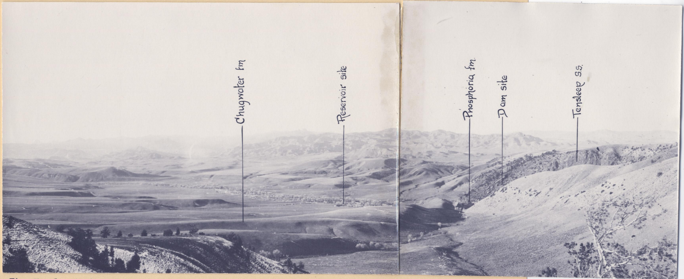
Fig. No. 1 - A view of the proposed reservoir and dam site looking northwest.
