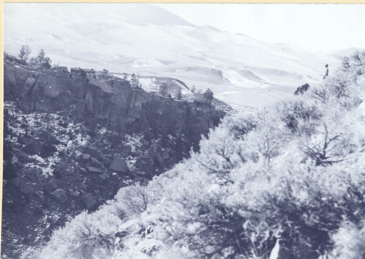
Fig. No. 2 - View of proposed dam site looking southwest. The man is standing on the line of the axis of the dam. The upper portion of the Tensleep sandstone is exposed on the south wall of the canyon.
