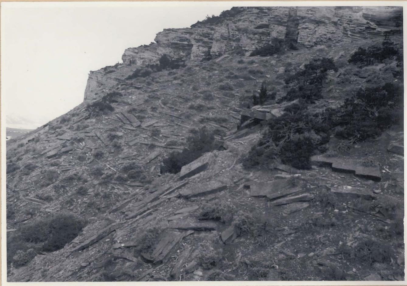
Plate VII. Talus slope north of the dam site showing blocks of resistant sandstone up to 6 feet long.
