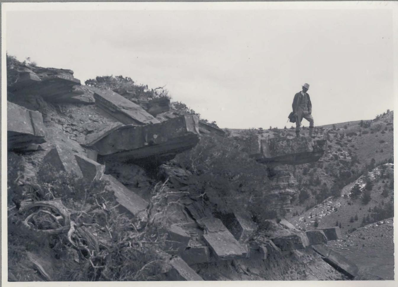
Plate VI. Resistant sandstone beds in the upper part of the Cody near the north abutment of the proposed dam.
