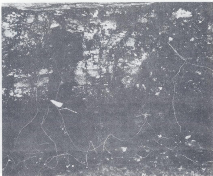
FIGURE 10. Coal face in the Rainbow No. 8 deep mine wired and ready for "shooting"
