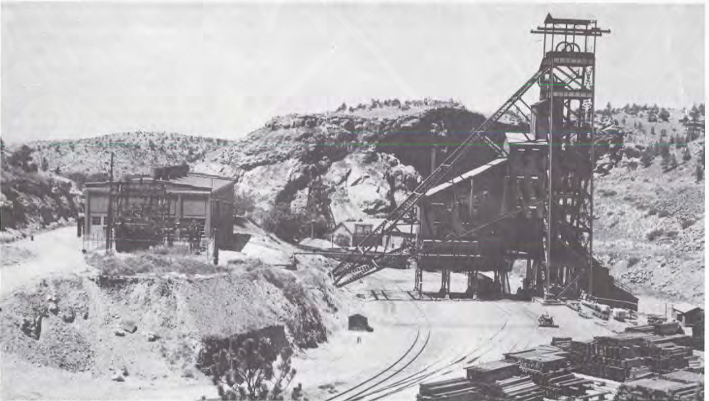
The production of iron ore from the Sunrise Mine in Platte County began in the late 1880's and led to the establishment of the town of Sunrise in 1902. The vein of iron ore—one of the purest iron deposits in the nation—extends over 35 miles from Guernsey north to Sunrise. (Wyoming Travel Commission Photo)
