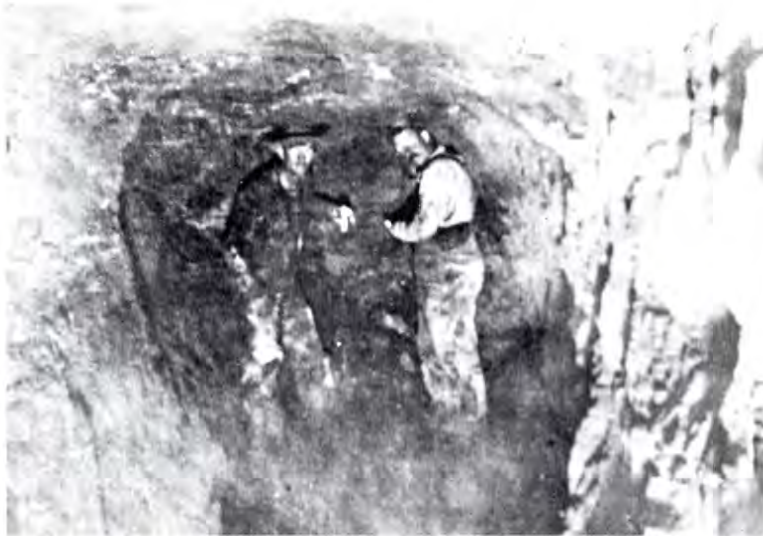
George Myers and John Irwin in Hidden Treasure Mine tunnel.
