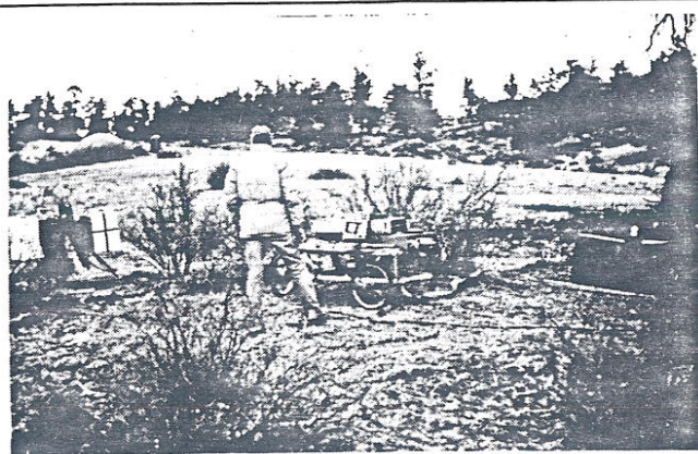
Figure 10. Microwave sounding on the Schaffer 3 pipe, Wyoming.
