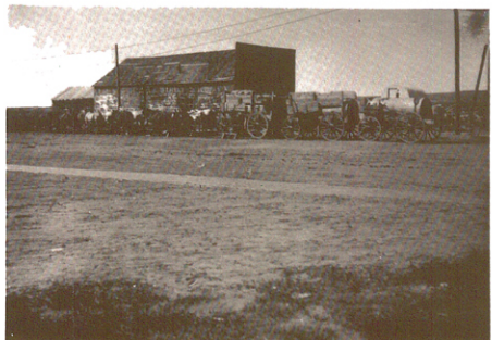
Oil was transported by wagon from Shannon Field to the refinery in Casper until the completion of a pipeline in 1911. A normal complement of wagons was pulled by 12 to 18 horses. Supplies and equipment were transported to the fields on the return trip. The trip was 60 miles one way and usually took at least two or three days. (Photo from University of Wyoming Petroleum History Center)
