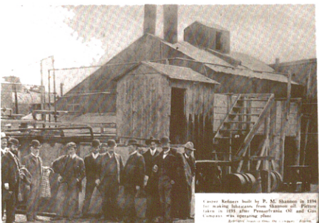
Shannon completed construction of this, the first refinery in Wyoming, in Casper in 1895. The refinery was quite small by today's standards, having a capacity of 100 barrels per day. Kerosene and lubricants were its first products, as there was no real use for gasoline at this time. (Photo from University of Wyoming Petroleum History Center)
