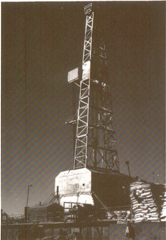
Parker Drilling Rig #112 contracted by Colorado Interstate Gas Company to drill the 1-6-36-88 Bldg Unit well in western Natrona County. This well was drilled to a depth of 20,850 feet in Waltman Field and completed in October 1979 in the Muddy, Dakota, Morrison, and Sundance, producing at the rate of 1,764,000 cubic feet of gas per day. (Photograph by compiler.)
