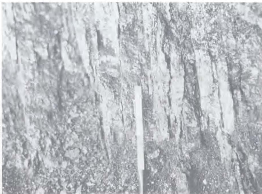
Figure 5. Closely spaced fracture zone immediately adjacent to a major fault (fractures strike parallel to the fault).
