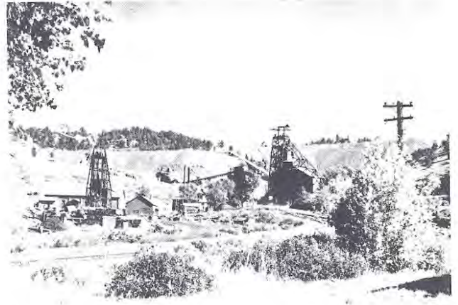
Figure 6: Colorado Fuel and Iron Company's Sunrise Mine in the Hartville uplift. The mine has a rated annual capacity of approximately 600,000 tons. Hematitic iron-formations are mined, and the ore is shipped to C.F.&I.'s blast furnaces located in Pueblo, Colorado (Hausel, 1978). Photograph by W. Dan Hausel, 1980.
