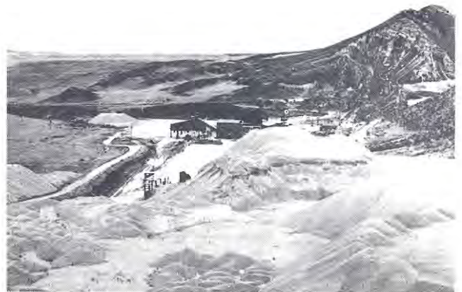
Figure 12: View of Great Western's Horse Creek property. While quarrying of this property began in 1912, underground methods are initiated in 1926. The limestone occurs in two steeply dipping ( 80^\circ\text{NE} ) massive beds that average 23 feet thick. The footwall is dolomite, and the hanging wall is hard massive red sandstone (Osterwald and others, 1966). More than four million tons of rock have been mined since 1912. Presently, five years of reserves are stored on the surface. Photograph by W. Dan Hausel, 1980.
