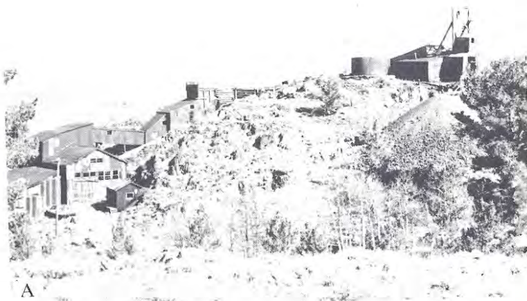
Figure 4: The historic (a) Duncan gold mine and mill was developed along (b) quartz veins in sheared metagabbro as were many of the important mines of the South Pass area (the quartz vein lies between the two drafted arrows immediately above the collapse breccia in the adit). Photography by W. Dan Hausel, 1978.
