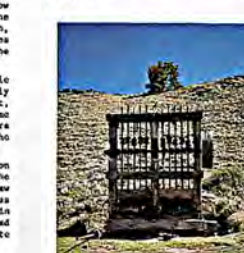
A battery of ten stamps south of South Pass City. Historic mine on the south bank of Willow Creek. Many early prospectors wrote about the constant thunder vibrating through the gold camps as these rock crushers pulverized gold ore. (Photo by W.D. Haeusel, 1983.)
