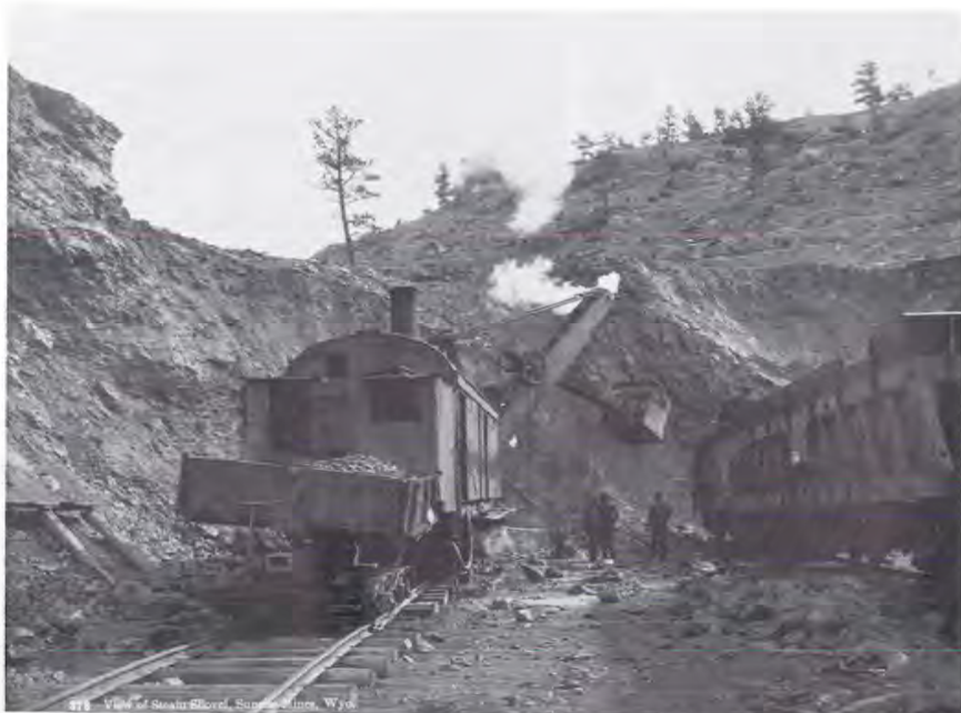
View of steam shovel operation, Sunrise iron mine, Platte County, Wyoming. This mine was visited by Hall in 1909 or 1910. (Photograph courtesy of AHC, J.E. Stimson collection.)
