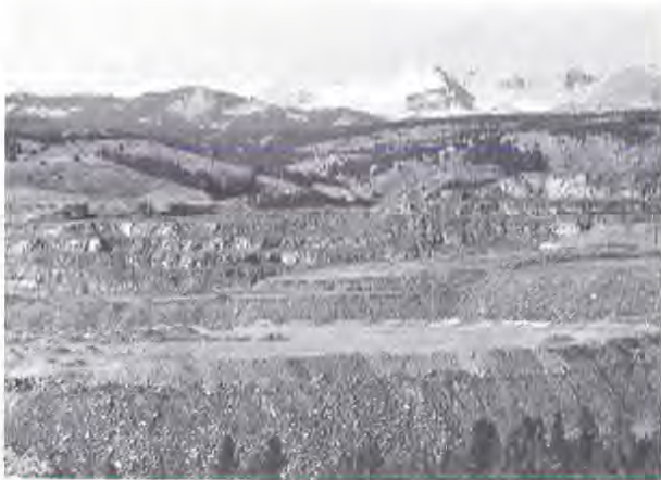
Figure 3. View of the Atlantic City iron ore mine looking west towards the snow capped peaks of the Wind River Mountains. At present, this is the only active mine in the Sweetwater District and annually mines an average of 5 million tons of taconite ore. Photograph by W. D. Hausel, Oct., 1977.
