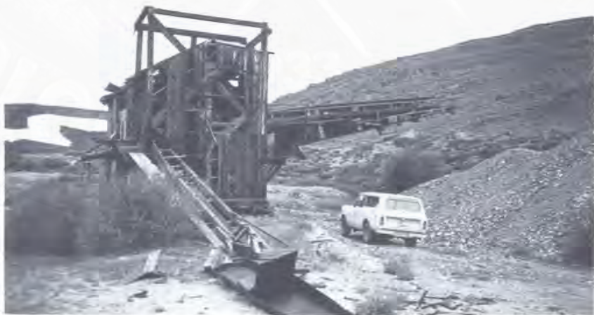
Figure 60. Remains of the E.T. Fisher washing plant used in the dredging of Rock Creek in the South Pass-Atlantic City district. The dredge operated from 1933 to 1941. (Photograph by W. Dan Hausel.)
