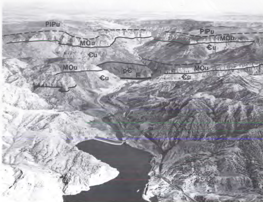
Figure 46. Aerial view across Boysen Dam into Wind River Canyon. Rock units include: Pc (Precambrian), Cu (Cambrian), MOu (Mississippian and Ordovician), PIPu (Pennsylvanian and Permian). Lower half of photo is a faulted complex of Paleozoic and Mesozoic rocks. F = Boysen normal fault. (Photograph by P.T. Jenkins, J. David Love collection.)
