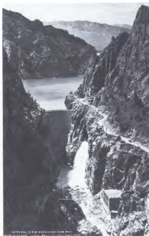
Figure 43. Buffalo Bill (Shoshone) Dam shortly after it was built. The dam is sited on Precambrian granite exposed on both sides of the dam. Steeply dipping Paleozoic rocks (Madison Limestone, Amsden Formation, and Tensleep Sandstone) are exposed on the cliffs across the reservoir. Madison Limestone can also be seen on top of Sheep Mountain on the skyline. (Courtesy of the American Heritage Center, University of Wyoming, Laramie.)
