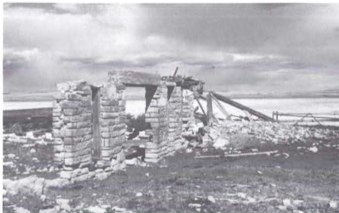
Figure 6. Abandoned epsomite processing plant at Rock Creek Lakes.
