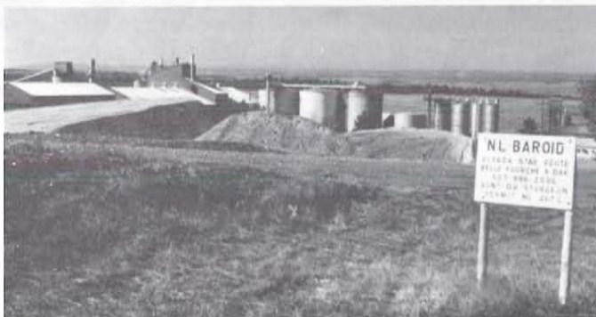
Figure 4. Baroid Drilling Fluids, Incorporated, bentonite mill at Colony, in northeastern Crook County. Bentonite from different pits is stockpiled outside of the mill and blended within the mill to produce bentonite products.
