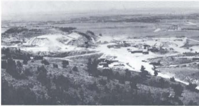
Figure 2. Air view (looking southeast) of the Guernsey Stone Company quarry one-half mile north of Guernsey. Aggregate from this quarry has been used for railroad ballast, other construction aggregate, and decorative aggregate.
