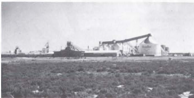
Figure 8. Rhone-Poulenc soda ash plant northwest of Green River. This plant refines trona to produce soda ash.
