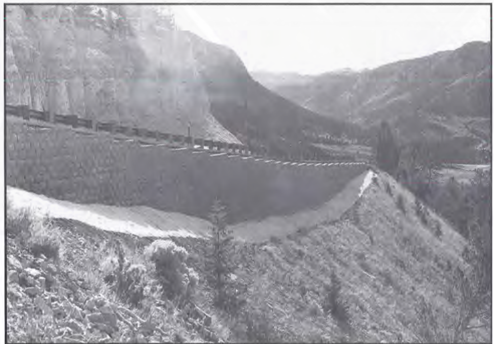
Figure 31. Completed geogrid retaining wall. Pilgrim Limestone exposed in roadcut to left. (Photograph by M.G.H., 1996.)
