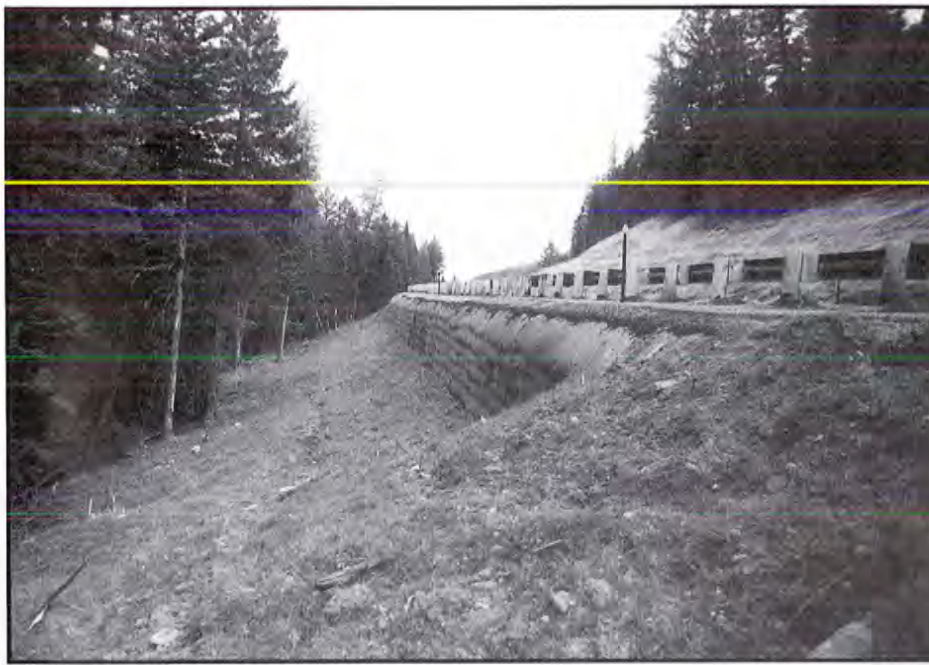
Figure 38. Rebuilt highway at Deadman Slide using geotextile wall covered with shotcrete to protect it from weather. (Photograph by M.G.H., 1992.)
