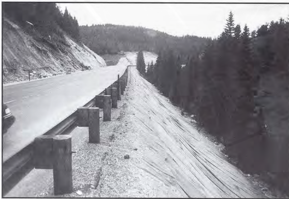
Figure 27. Geogrid reinforced fill along road through Paint Creek. View is to west. Note rockfall mesh installed on unstable backslope on left side of road. (Photograph by M.G.H., 1996.)
