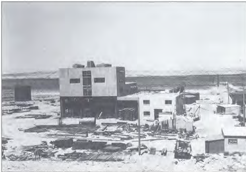
Figure 11. Construction of FMC's soda ash plant, 1952. (Photograph from Sweetwater County Historical Museum, Green River, Wyoming.)
