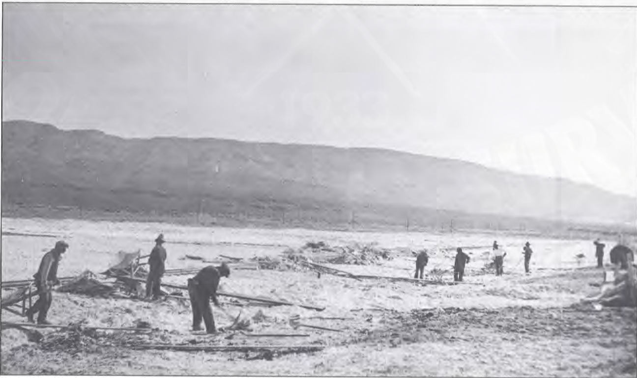
Figure 7. Workers using picks and shovels to harvest the crude trona from the evaporation ponds at Owens Lake, California. (Photograph from Eastern California Museum, Independence, California.)
