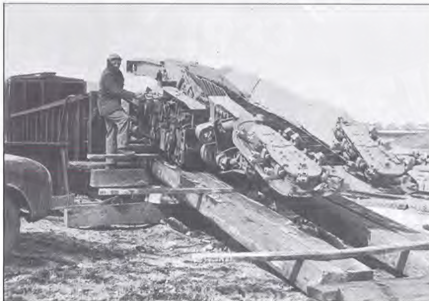
Figure 10. Delivery of a Goodman 665 ore loader to Westvaco Chemical Corporation, 1949. (Photograph from Sweetwater County Historical Museum, Green River, Wyoming.)
