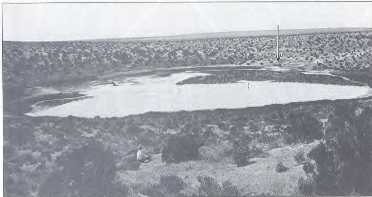
Figure 2. Little Soda Lake. One of the members of the King Expedition is in the middle-left foreground. The arrow points to a small wooden structure that could have been used to store crude soda. Photograph taken by Timothy O' Sullivan sometime between 1867 and 1872. Compare with 1909 photograph on page 10. (Photograph from the National Archives.)
