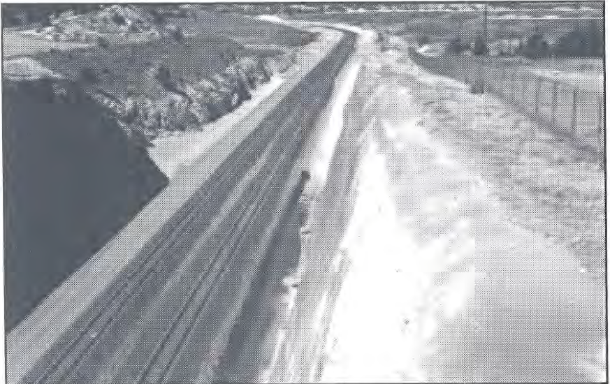
Figure 18. A double-tracked cut has recently replaced the Burlington Northern/Santa Fe's single-track tunnel east of Guernsey, Wyoming.
