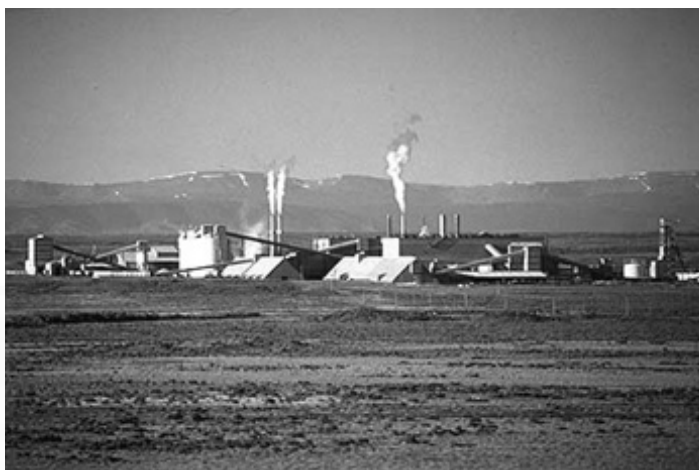
Figure 24. Solvay Minerals soda ash refining plant west of Green River. The structure at the right of the photograph is the headframe that provides access to the mine workings 1600 feet below the surface. (Photograph by Solvay Minerals, 1998.)
