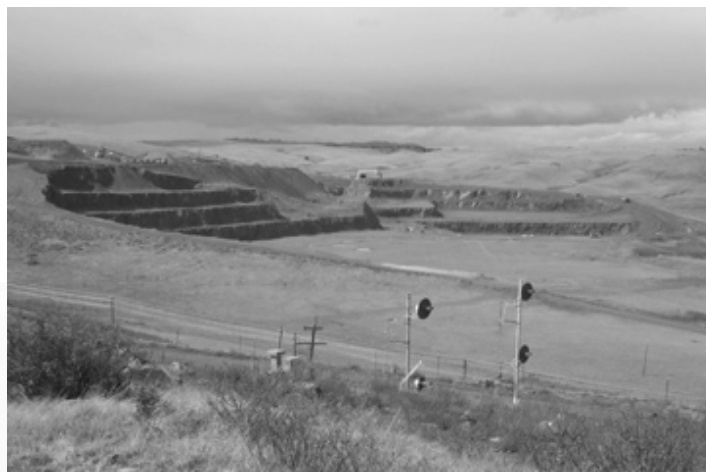
Figure 21. Martin Marietta Materials (formerly Meridian Aggregates) granitic aggregate quarry, Granite Cañon, Wyoming, September 28, 2000. Train above benches, upper left center, for scale.
