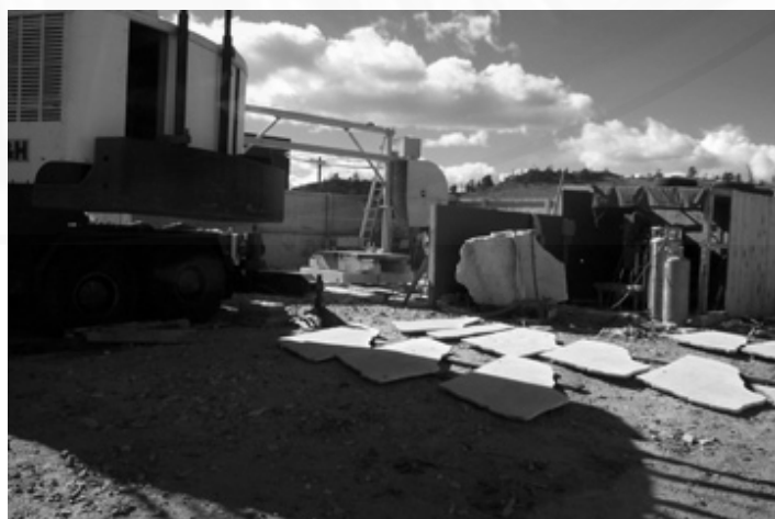
Figure 23. Slabs processed by Raven Quarries at the quarry site in Albany County. Wireline saw (with ladder and circular drive shield) in background, October 13, 2000.
