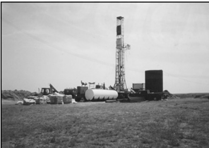
Figure 39. Water Systems Drilling Inc. rig on site at the Mule Creek Junction water well.
