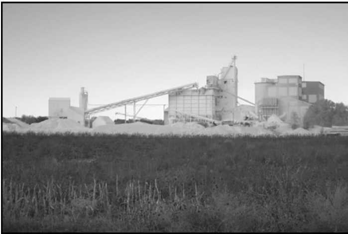
Figure 23. Imerys Marble processing plant near Wheatland.
