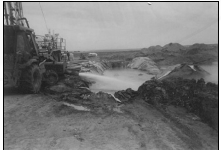
Figure 40. Hot water (160°F) from the Madison Limestone being produced during testing of the Mule Creek Junction well.
