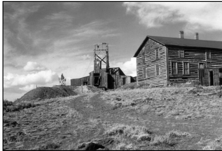
Figure 31. Duncan mine headframe and mine dump.
