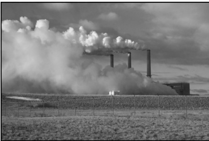
Figure 25. Basin Electric's Laramie River power plant northeast of Wheatland. Limestone from the Hartville quarry is used in emissions control, primarily to lessen sulfur dioxide emissions. Most of the emissions seen here on a cold January morning are water vapor. This plant uses around 50,000 short tons of limestone per year for emissions control.
