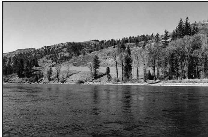
Figure 44. View of completed Elbow Slide project northward from the Snake River, showing the face of the MSE wall (the blank featureless area behind the trees) and the new highway. Note powerline near skyline which traverses the large landslide mass above roadway.
