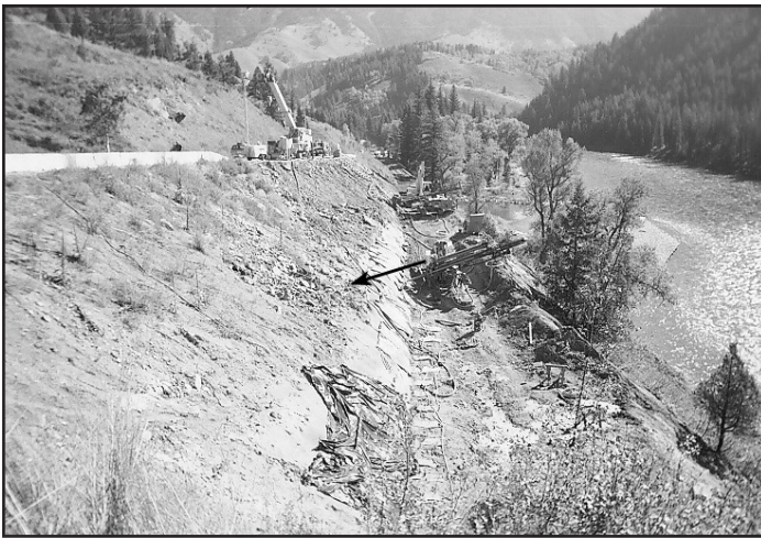
Figure 38. Construction of upper soil nail wall at Elbow Slide (view to east). Rig is drilling holes for placement of soil nails in wall (arrow shows orientation of soil nails). Grouting and nail placing equipment is just beyond the rig.
