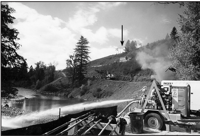
Figure 42. Construction of lower soil nail wall at Elbow Slide. Soil nails in foreground are ready for placement by grouting equipment to right. Note the tour bus on highway (below arrow).
