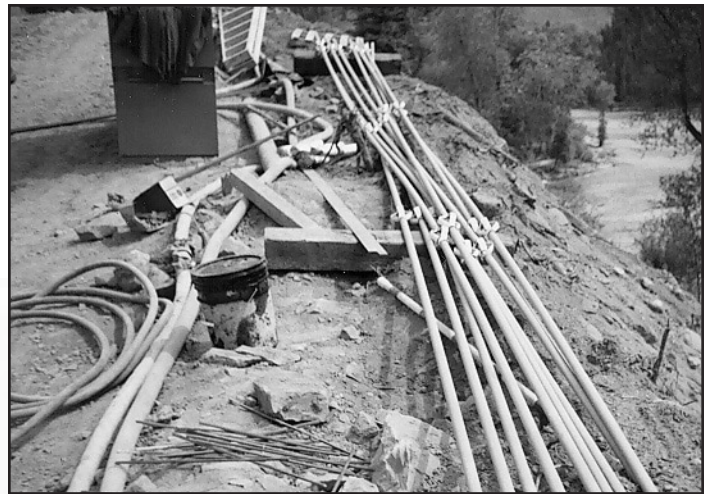
Figure 39. Soil nails with centralizers ready for placement in nail wall. These are 30 and 40 feet long, and some were instrumented with strain gauges along their length.
