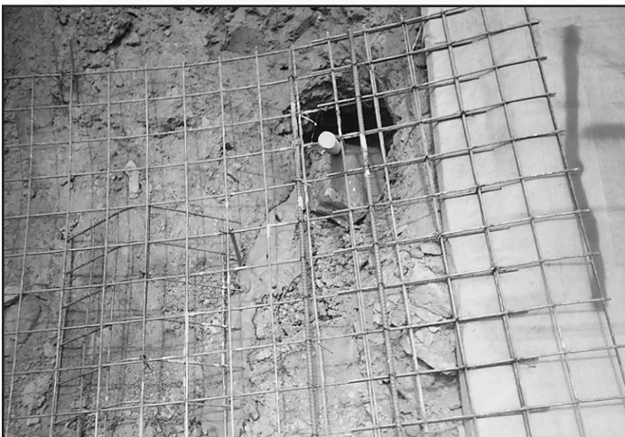
Figure 40. A completed soil nail hole after grouting into place; welded wire fabric is ready for attachment to the nail.
