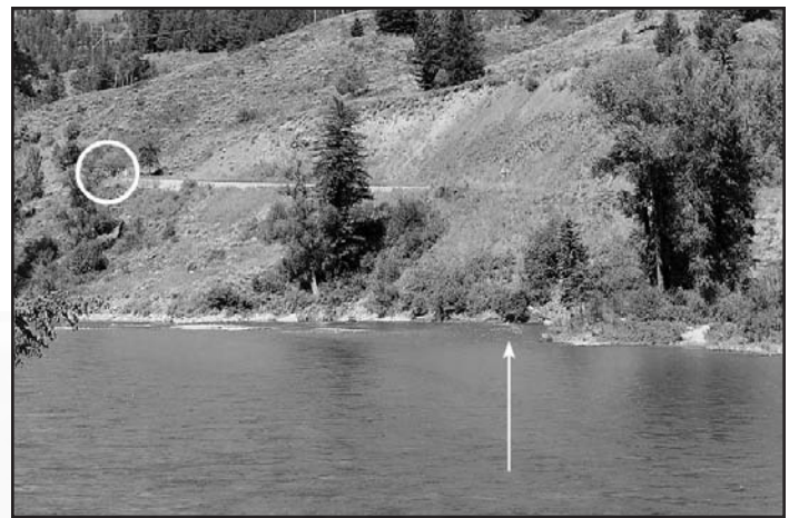
Figure 36. View from the river of Elbow Slide project area before construction showing active erosion of slope (arrow) by Snake River channel. Circled area in left center is a WYDOT carryall with several persons nearby. Note hummocky topography of large landslide area above circle.
