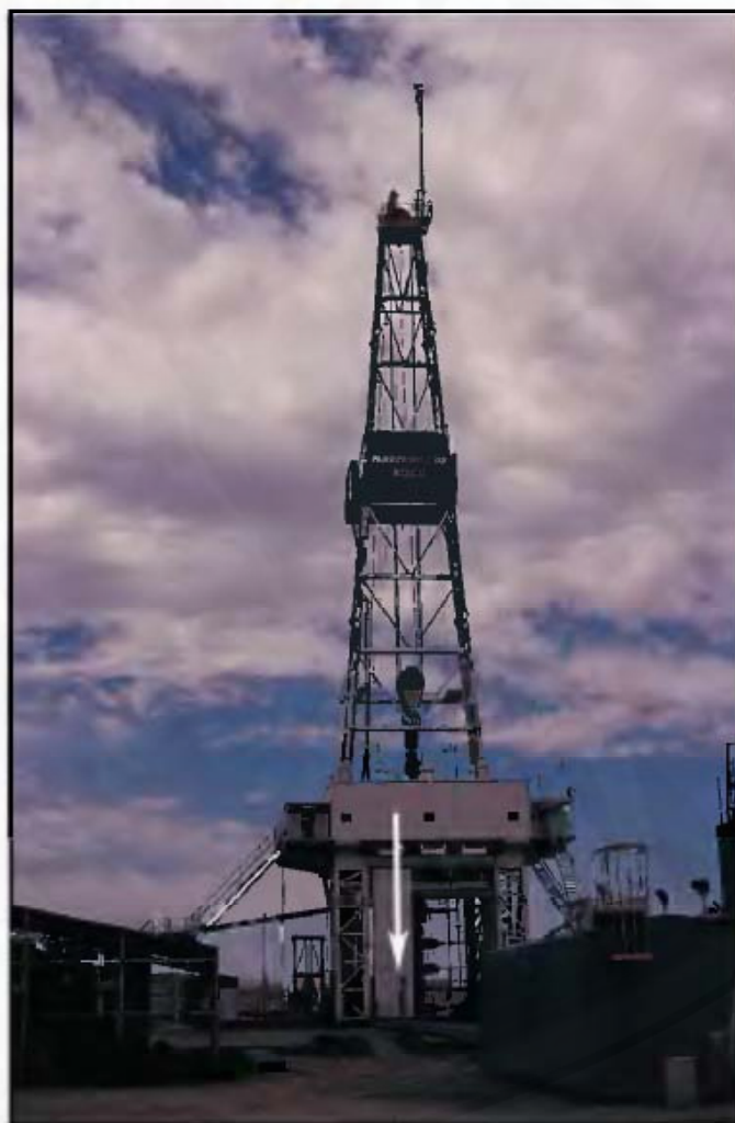
Figure 4. Parker Brothers' (now Unit Drilling's) Rig No. 201 on location at a Madden deep test. The ultra-deep rig is one of the largest land-based drilling rigs in the world, capable of drilling to depths of 30,000 feet. Arrow points to man standing at ground surface, some 50 feet below the rig floor. Photograph by Rodney H. De Bruin, summer, 1996.
