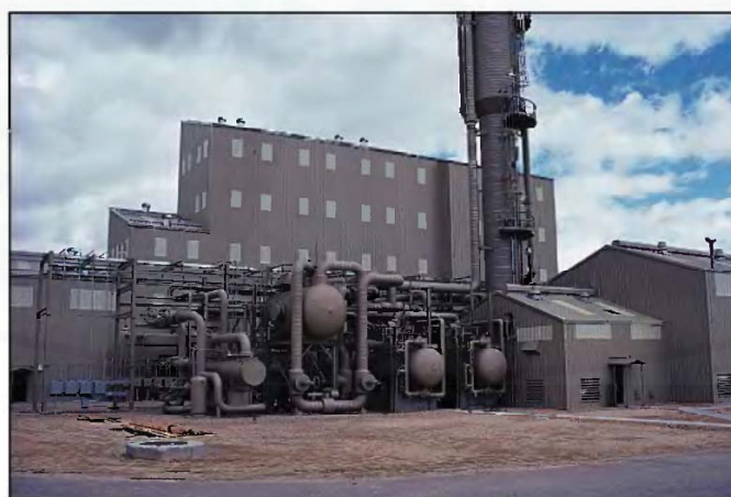
Figure 8. The carbon dioxide processing plant at Bairoll recovers and recycles carbon dioxide (from La Barge) that is injected at Lost Soldier/Wertz Oil Fields. Photograph by A.J. VerPloeg, Wyoming State Geological Survey.
