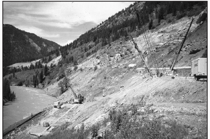
Figure 31. Construction of upper and lower RMP walls required temporary cut and fill benches to accommodate equipment. Another RMP wall was installed west of these two walls 39.4 feet (13 meters) below the roadway to stabilize the slope beneath an MSE wall.
