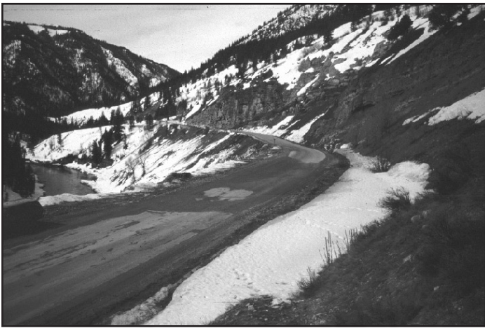
Figure 27. View to southwest across Blue Trail Slide from near roadway level before construction began. Snake River in center left of photograph. Dark area in the road (center of photograph) indicates where the road had been patched repeatedly over the years across the active part of the slide.
