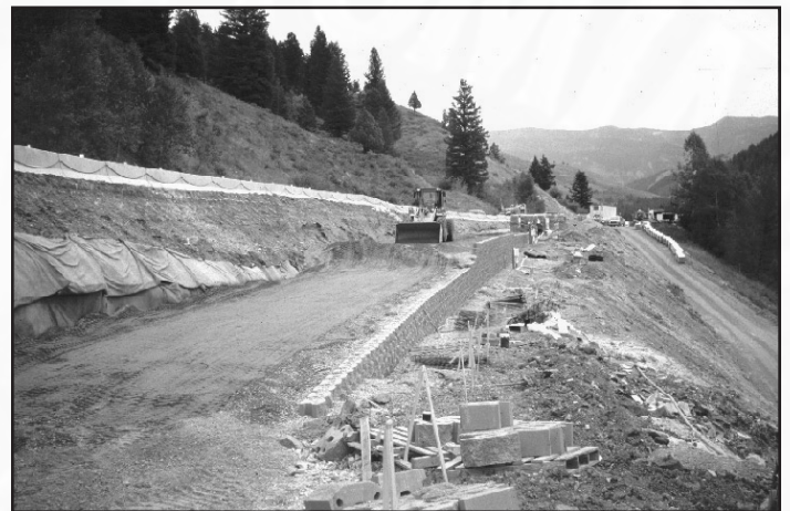
Figure 35. Construction of the MSE wall used geo-grid supported backfill tied into keystone block facing. This wall was built up to the height of the roadway at the base of the concrete barriers.
