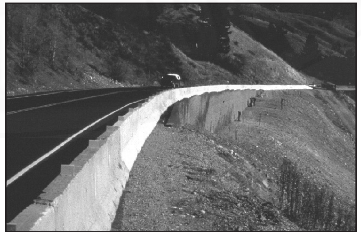
Figure 36. Completed highway reconstruction over Blue Trail Slide viewed to east. Note MSE wall with inclinometers and other instruments to measure and monitor stresses and loads in the slide and on the anchors and micropiles.
