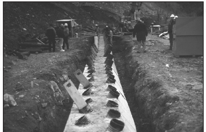
Figure 32. Concrete cap beam showing position of battered micropiles. Tieback anchors were then installed at a shallower angle into the bedrock and attached to the cap beam.
