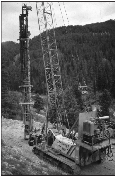
Figure 33. Drilling rig suspended on a crane was used to drill holes and install micropiles and tieback anchors.
