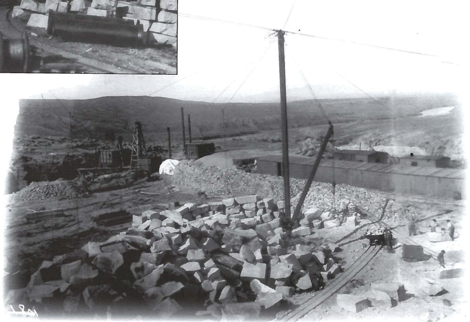
Figure 66 (right). The cement was prepared in sheds (long buildings on right) and transported to the mixing houses near the canyon's edge where it was combined with sand and aggregate to make concrete or moved to the dam to be used as mortar. Part of the quarry is seen in the foreground. Photograph by W.C. Knight, courtesy S.H. Knight Collection, American Heritage Center, University of Wyoming (used with permission).
