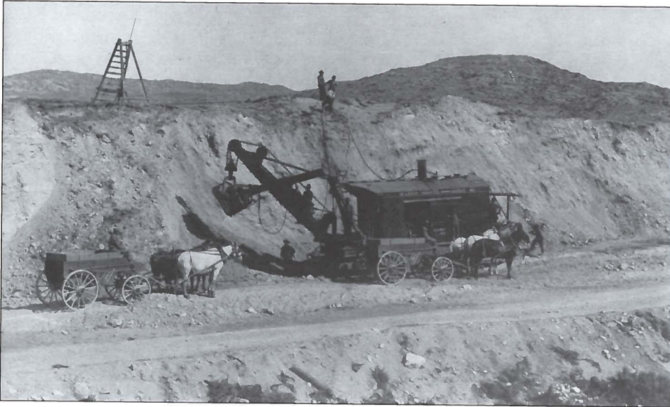
Figure 70 (left). A steam shovel was used at the construction site only after the main part of Pathfinder Dam was completed.
