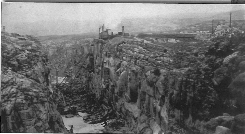
Figure 60 (left). Early part of construction of Pathfinder Dam after river was diverted through tunnel.
