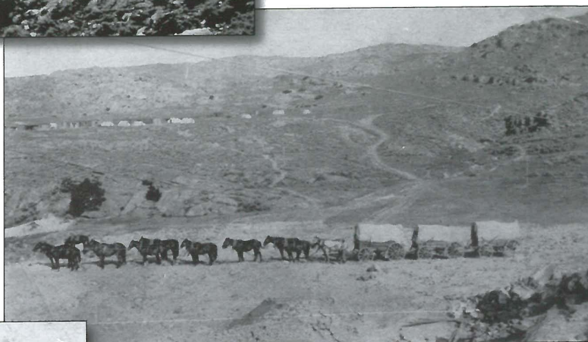
Figure 73 (right). A closer view of the wagon trains used to haul supplies to Pathfinder. Note the white tents in middle background used to "house" construction workers.
