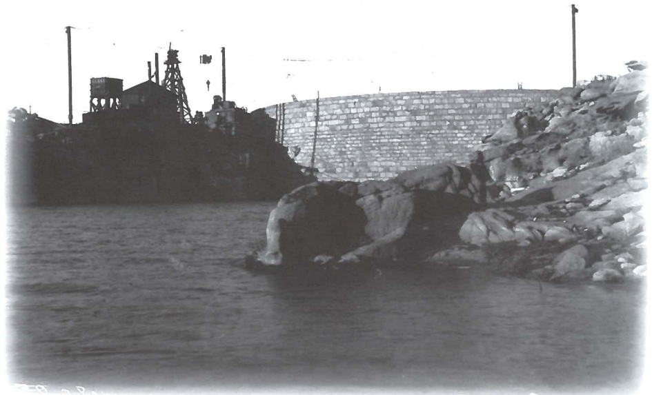
Figure 71 (right). The upstream end of completed Pathfinder Dam. Because the height of the dam exceeded the height of the canyon walls, a retaining dike had to be constructed south of the dam and a spillway system built on the north end of the dam to handle excess water in wet years.
