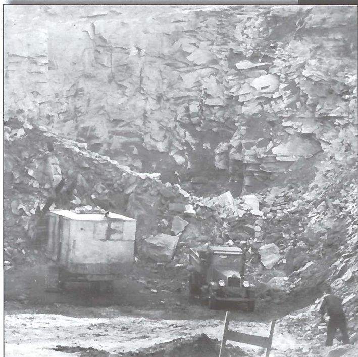
Figure 22 (left). Excavating the foundation and canyon walls for Alcova Dam.
