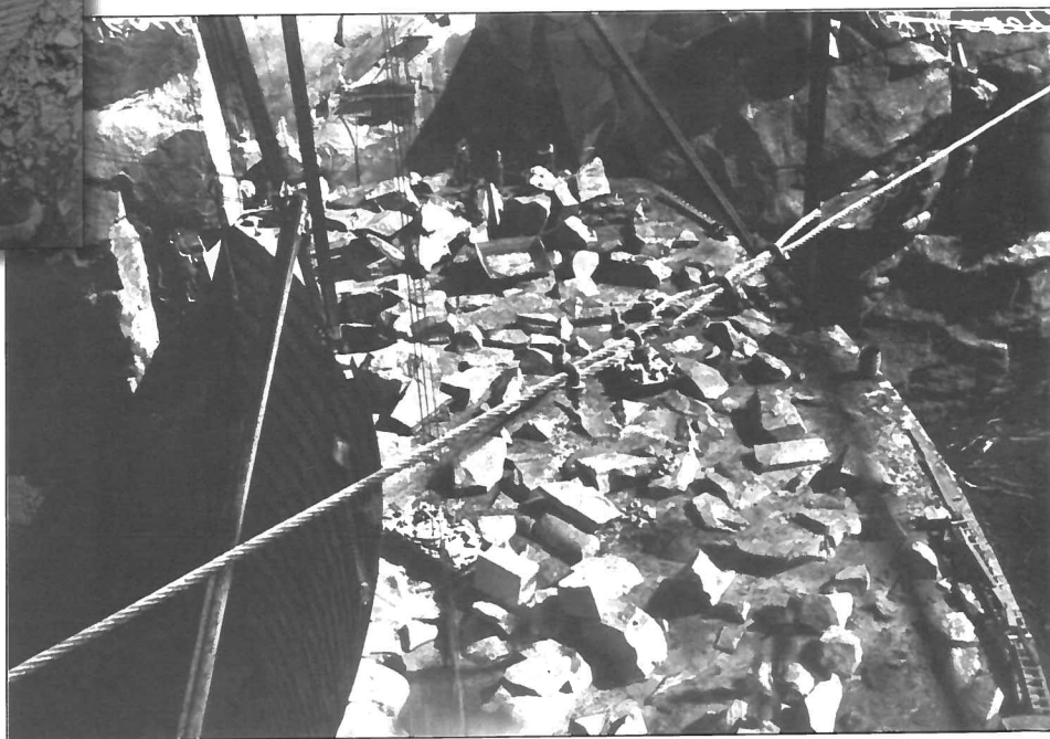
Figure 68 (right). Pathfinder Dam, circa 1909, showing placement of granite blocks and rubble. Photograph by W.C. Knight, courtesy S.H. Knight Collection, American Heritage Center, University of Wyoming (used with permission).
