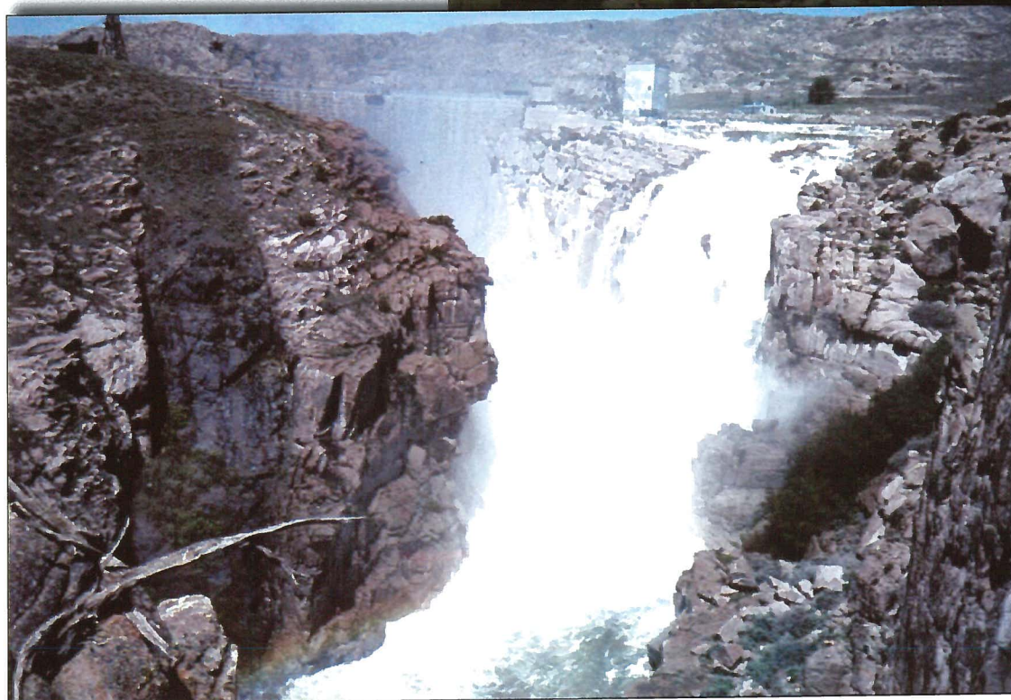
Figure 78 (below). The south wall of Fremont Canyon just below Pathfinder Dam contains a black diabase dike that intrudes Precambrian granite. The dike is the dark vertical band on the left side of the photograph. In wet years when Pathfinder Reservoir is completely full and not enough water can be run through Fremont Canyon Power Plant, the dam is allowed to "spill" around its north end, creating a very impressive waterfall into the canyon below.
