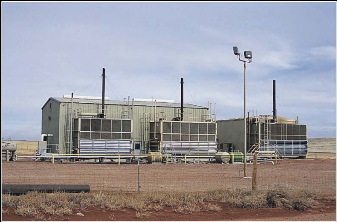
Figure 11. Compressor station where coalbed methane is compressed before transport through a pipeline.
