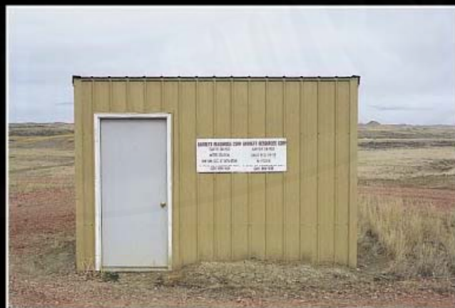
Figure 10. Coalbed methane facility, which houses equipment that measures production from a number of coalbed methane wells.
