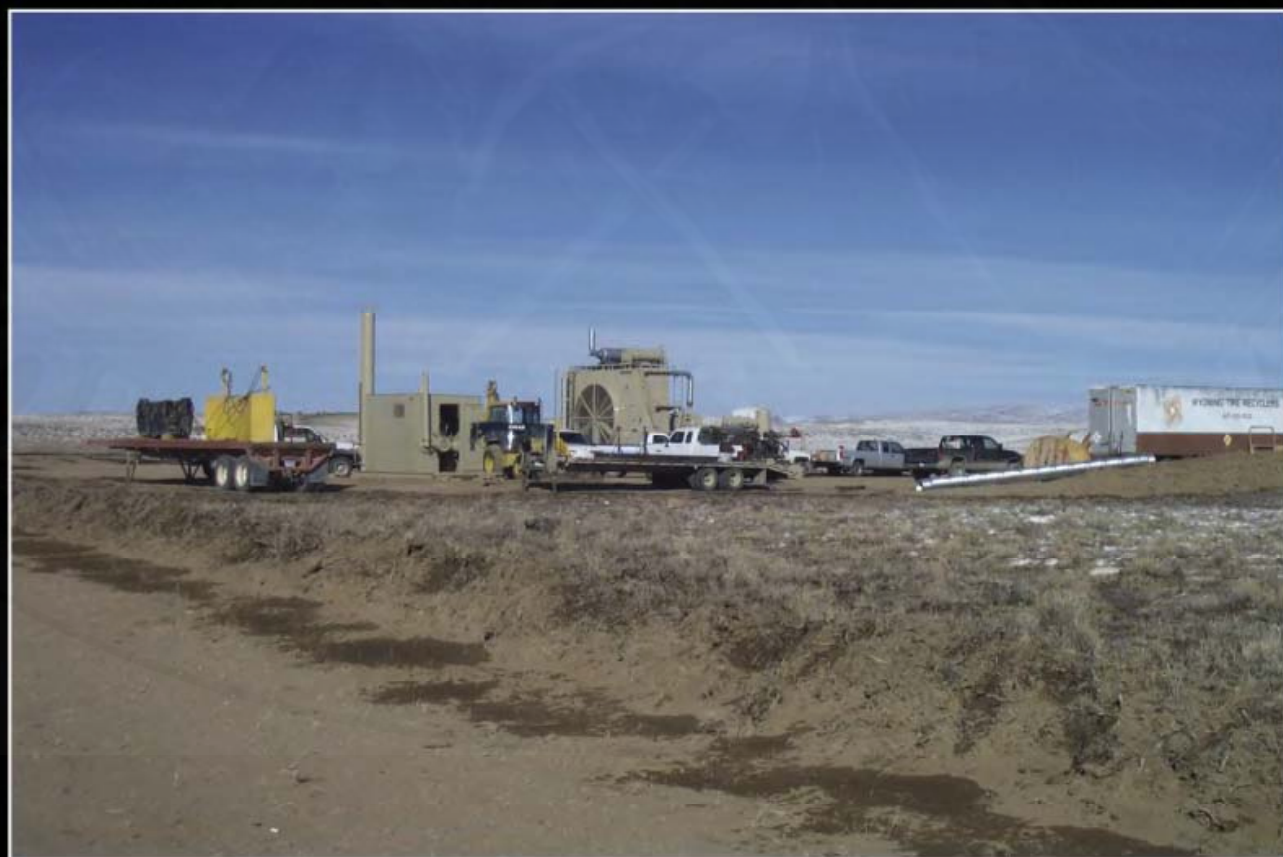
Figure 17. In-field coalbed methane compressor facilities (under construction) in the southeastern part of the Green River Coal Field. A natural gas powered unit (center, with cooling fans) provides power to the facility.
