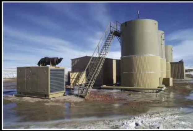
Figure 12. Water injection facilities operated by Petroleum Development Corporation north of Baggs. Tanks store water produced from several coalbed methane wells, which is then reinjected into the subsurface by pumps (housed in building behind stairway) powered by portable unit (on left).
