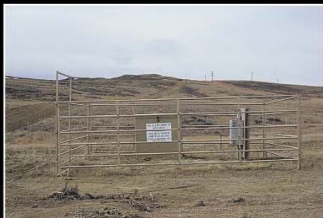
Figure 9. A single coalbed methane well south of Gillette. As shown here, the surface equipment for many producing wells is enclosed in a small fiberglass or aluminum shell; other wells contain no structures and are simply wellheads enclosed by a fence.
