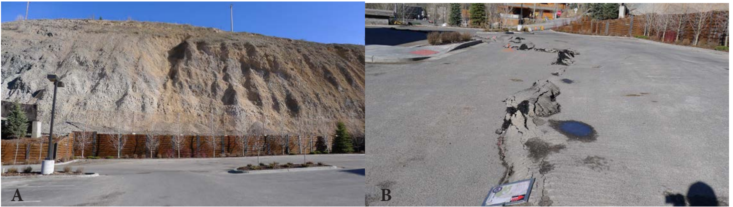
Figure 2A. View from the Jackson Walgreens parking lot, looking directly upslope toward the body of the landslide. B. The movement or motion of the landslide caused the asphalt to buckle and deform in the parking lot. Photo by Martin Larsen, WSGS, April 16, 2014.
