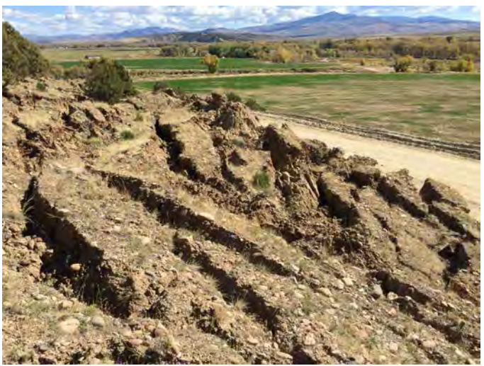
Figure 5. Recent landslide along Carbon County Road 702.
