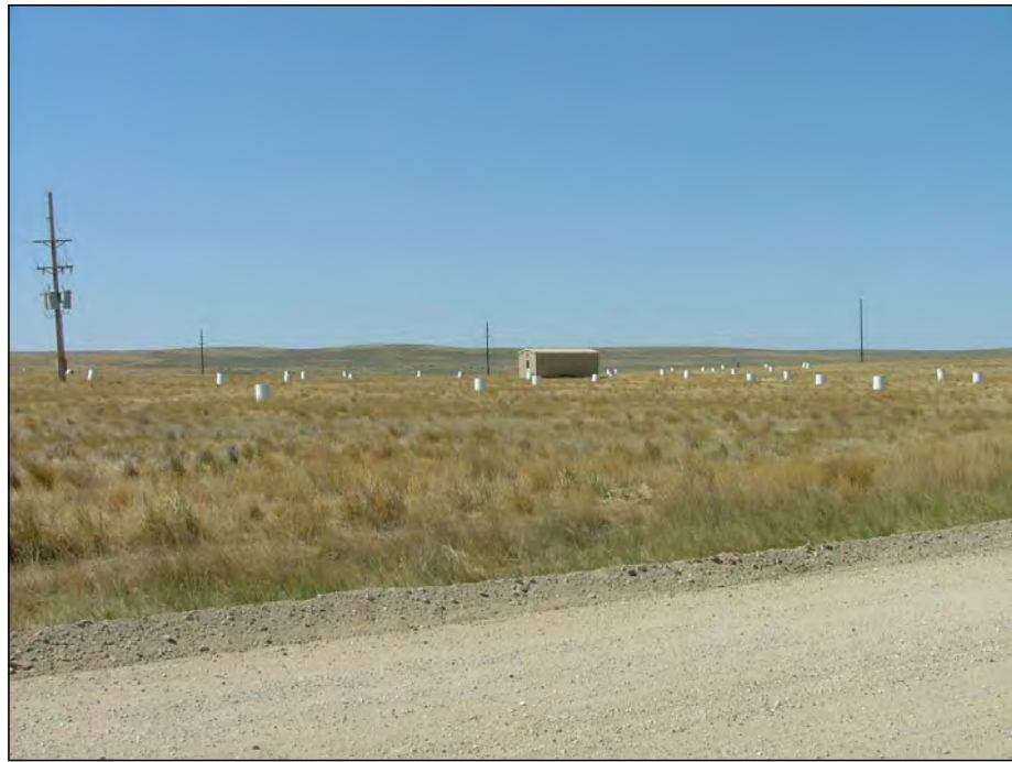
Figure 16. Header house and well heads in an ISR field at the Smith Ranch-Highland mine operation in Converse County, Wyoming. (Photo by Robert W. Gregory, 2006).
