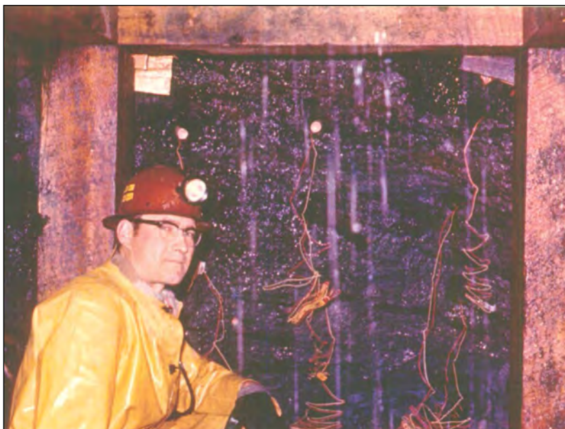
Figure 13. A miner prepares for blasting in the underground mine at Shirley Basin (circa 1960). Surface pits eventually succeeded underground operations at Shirley Basin and currently plans are in place for in-situ recovery operations sometime in the next few years. (Photo courtesy of R.V. Bailey).
